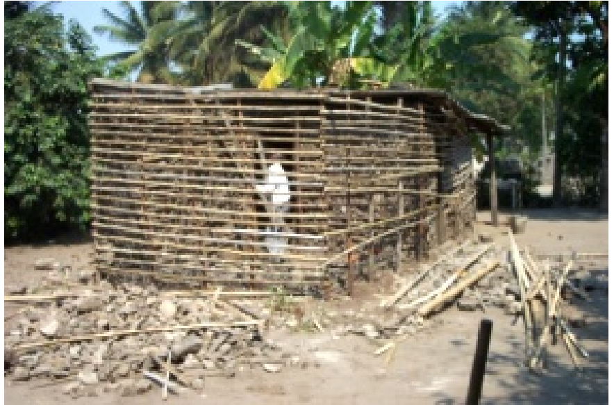
Pictured is Ps Pereira in his house, during the first day of re-construction. The house would be no larger than an average bedroom in Australia or America. The walls are made with bamboo and stone, the roof with plastic and reed. Ps Pereira lives there with his wife and seven children!
