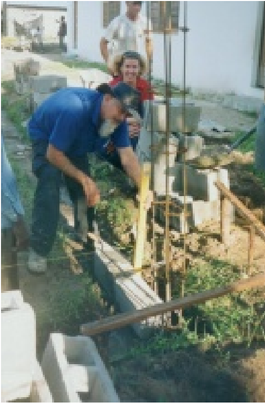
Macca laying the first blocks laid on the new classrooms
