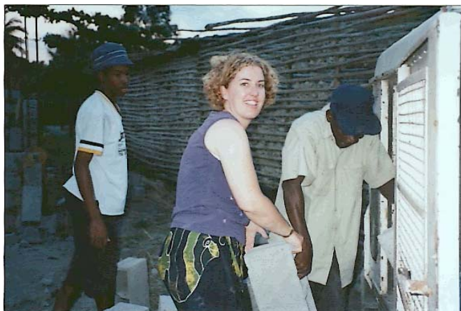
Emma helping with construction of the MozOutreach School
