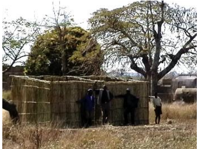
Justinio and Palestina's new house under construction in Umpala
